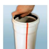
**3-** Apply liquid soap or a suitable lubricant to the gasket.
