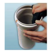
2- Place the gasket to the already cleaned nest putting the flat side of the gasket on the nest's surface and the dome of the gasket to face inner side of the pipe.
