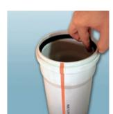
**4-** Also clean and apply a suitable lubricant to the surface of the connecting pipe or fitting which will be fixed to the related pipe.
